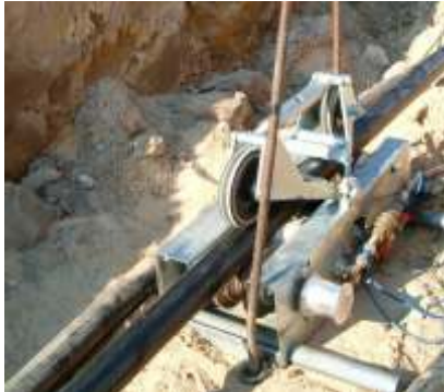
BKS 400 in a trench
